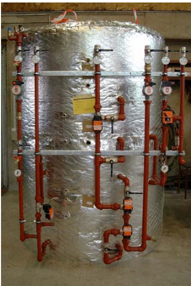
Aluminum-coated glass wool mats with mesh grid
