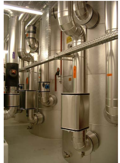
Special insulations (e.g. aluminium-coated or for cold storage)
