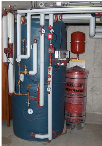
Glass wool or foam (fire classification III or V) with plastic shell
