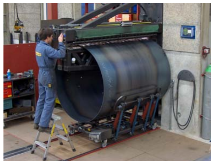
The lengthwise weld is performed automatically
