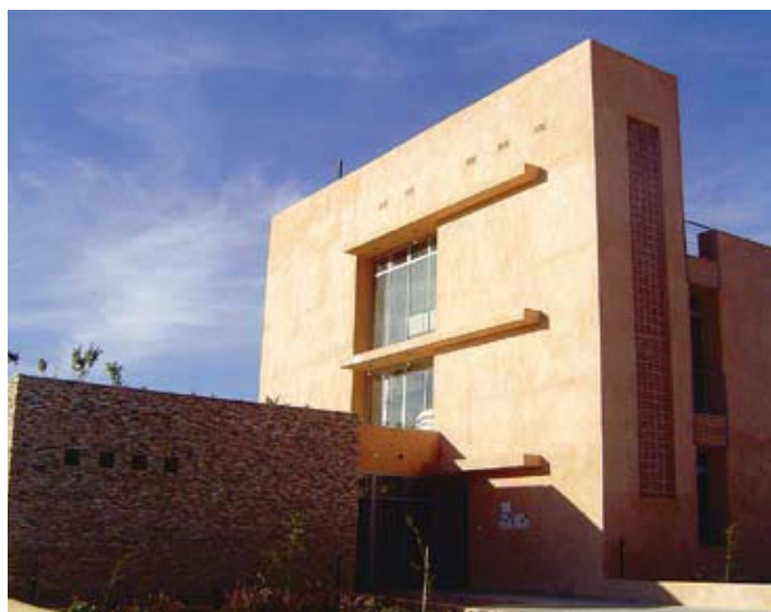
On the Aqaba Residence Energy Efficiency (AREE) Building in Jordan 38 m 2 of vacuum tube collectors provide energy for both solar heating and cooling.
