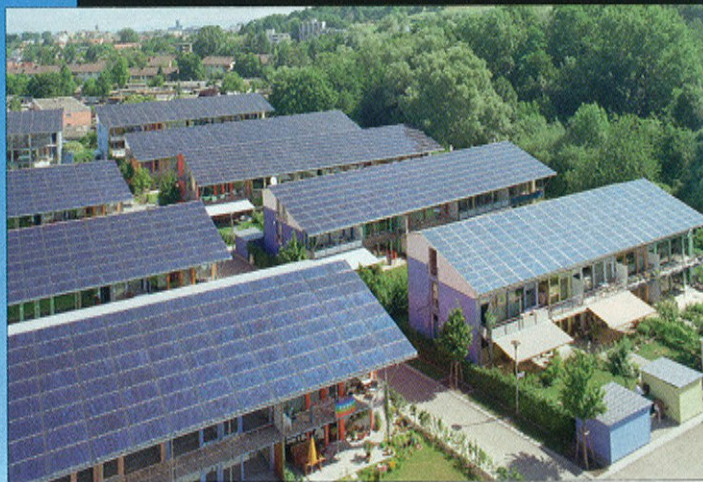
Photo 5a: Plus-energy houses in Freiburg, South Germany: Architect Rolf Disch built a whole community of 58 super-insulated houses with PV installations on the south-facing roofs.
