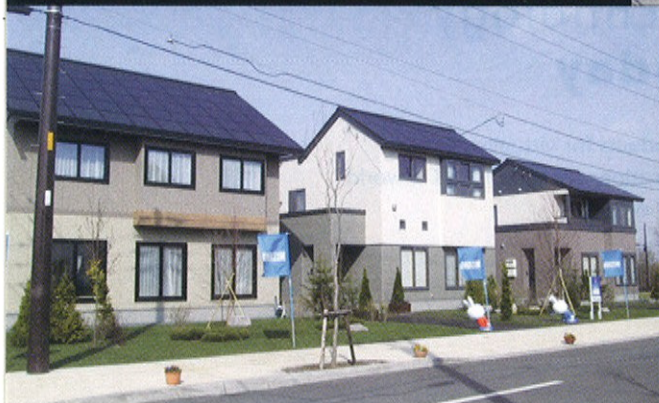
Photo 10: Solar power installation as a trademark: Suntech-MSK integrated a 1 kW p PV system into every roof in this Japanese solar housing community in Hokkaido. Photos (2): Suntech-MSK
